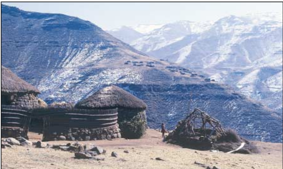
The winters can be harsh, but the Basotho plan their huts to minimise the effects of low temperatures through proper orientation of the huts and use thatched roofs.
