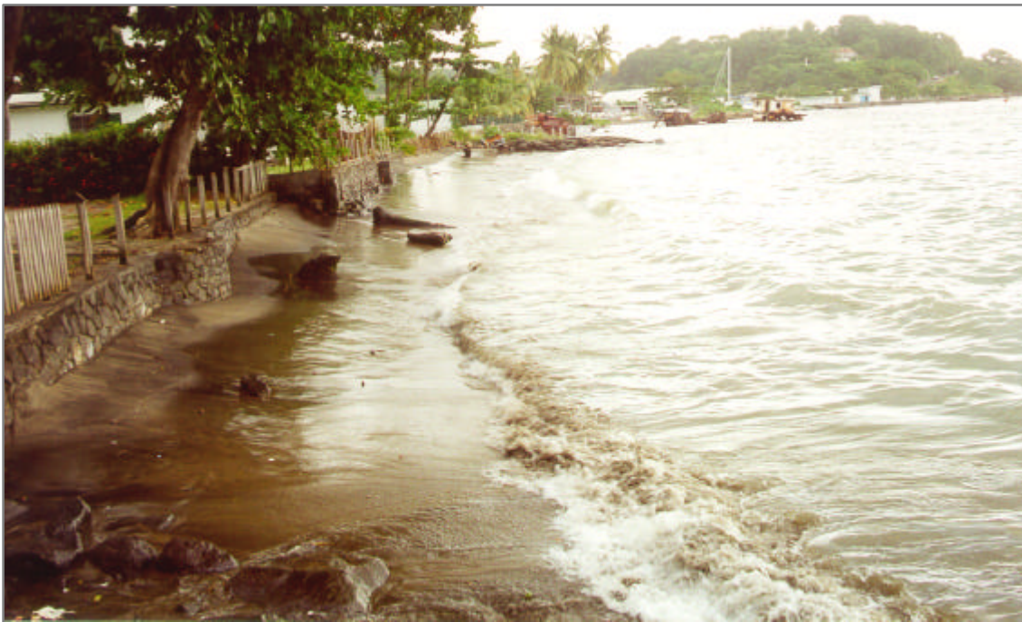
Photograph 4-6: Seawall along Villa Beach
