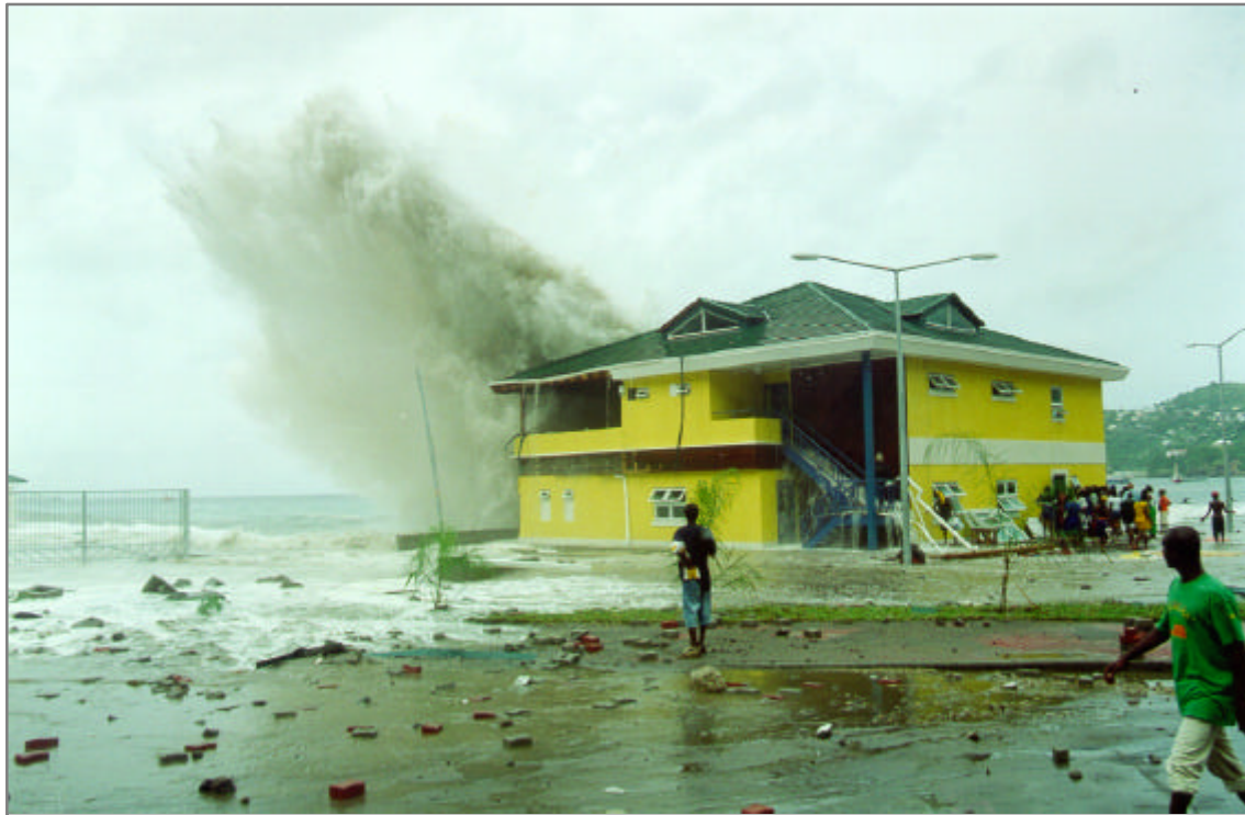
Photograph 4-3: Storm Surge over new Cruise Ship Terminal
