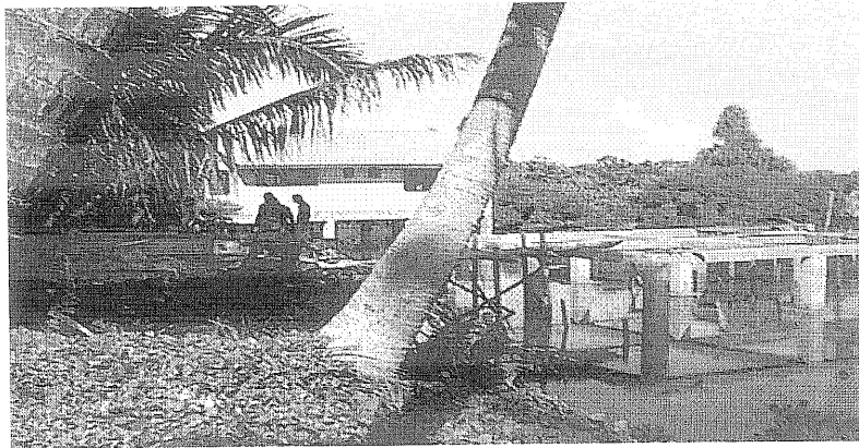
Photo 6: House build on fish pond - Funafuti
